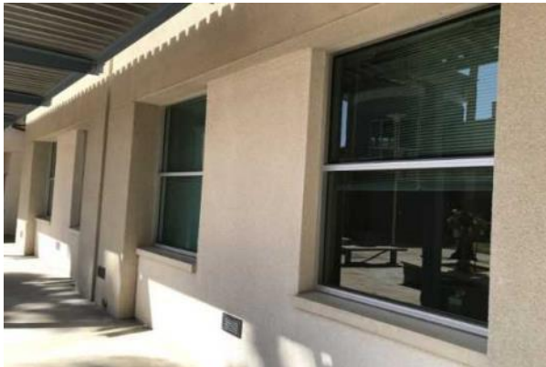
#9 EXTERIOR METAL WINDOWS, STUCCO FACADE
