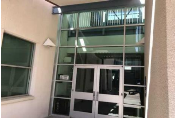
#7 EXTERIOR FULLY GLAZED DOOR, STOREFRONT GLASS
