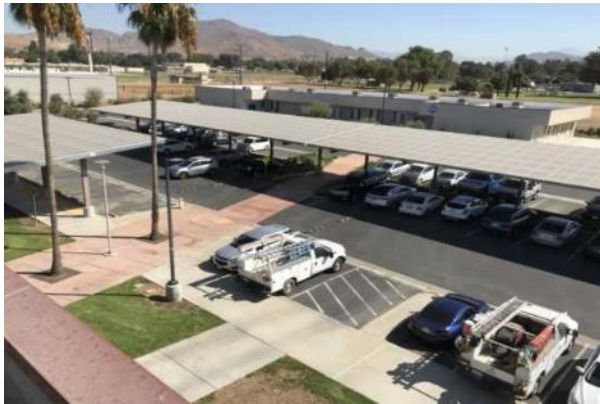
#57 PARKING LOT STRIPING, SOLAR PANEL CAR PORT
