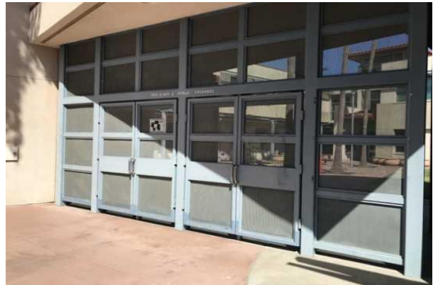
#10 EXTERIOR METAL MESH DOORS AND WALL
