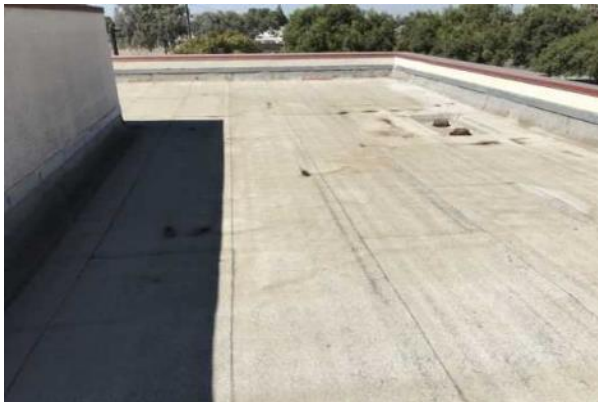
#11 MODIFIED BITUMINOUS ROOFING
