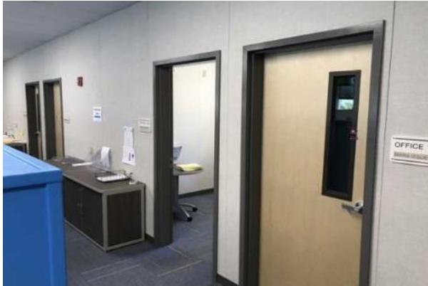
#25 PARTIALLY GLAZED WOOD DOOR, FIBERBOARD WALL
