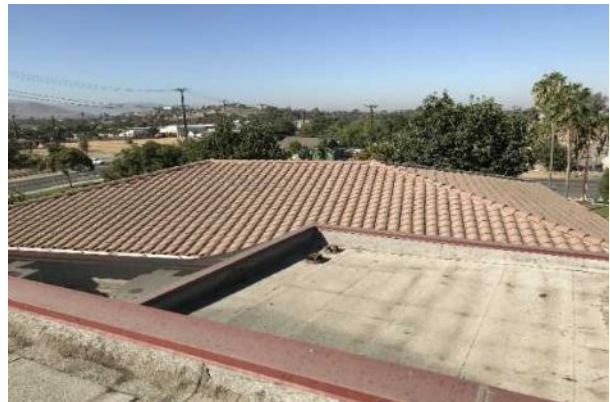
#12 CLAY TILE ROOFING
