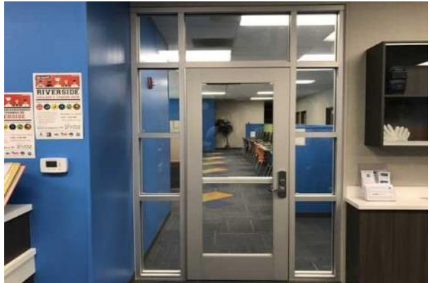
#24 INTERIOR METAL FULLY GLAZED DOOR
