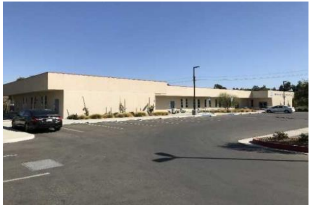
#58 PARENT CENTER BUILDING
