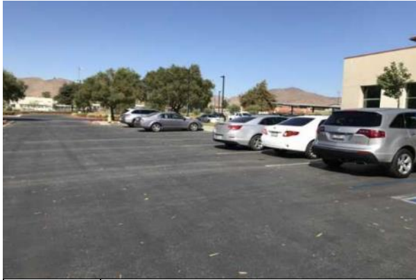
#55 ASPHALT PARKING LOT
