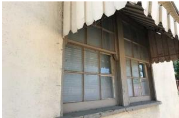
#6 STUCCO FACADE, EXTERIOR WOOD WINDOW
