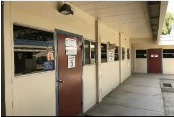
#7 METAL FACADE, EXTERIOR STEEL WINDOW
