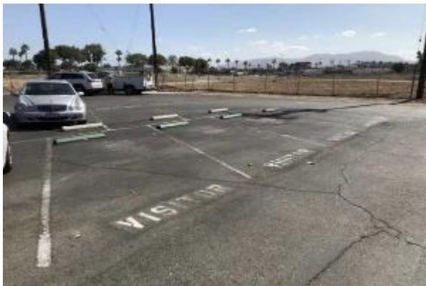
#35 ASPHALT PARKING LOT
