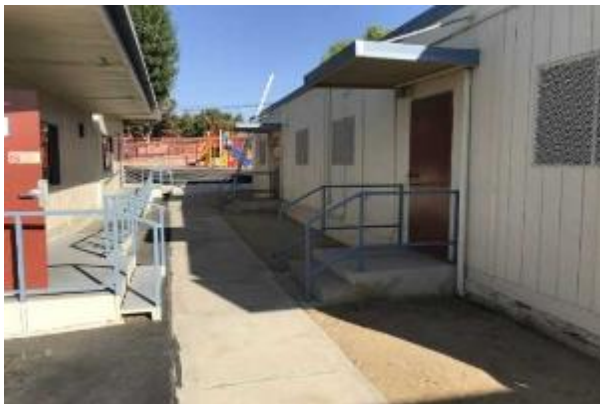
#5 WOOD FACADE, EXTERIOR RAMP AND STAIRS
