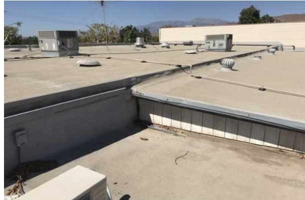
#22 PRIMARY ROOF OVERVIEW
