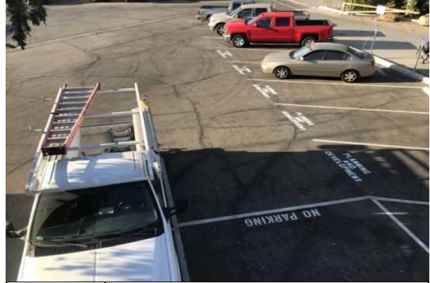
#44 CRACKING ASPHALT
