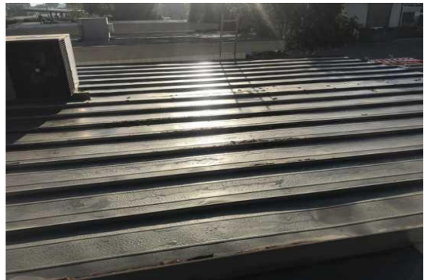
#42 SECONDARY ROOF OVERVIEW
