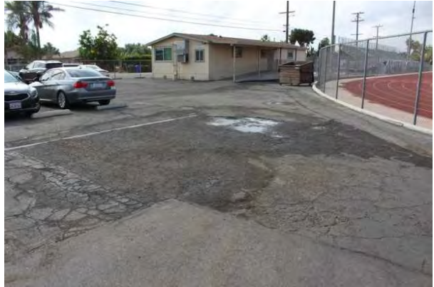
#38 PARKING LOTS, ASPHALT PAVEMENT
