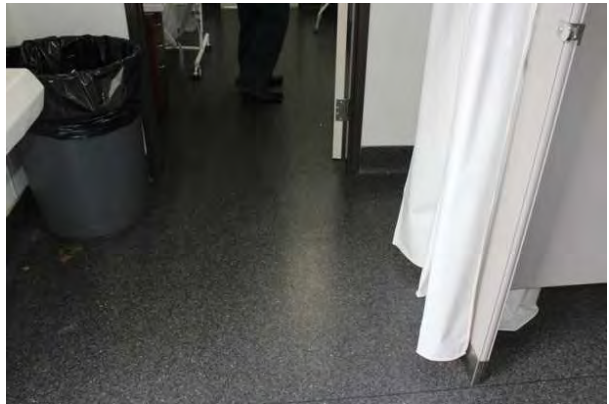
#16 INTERIOR FLOOR FINISH, LINOLEUM
