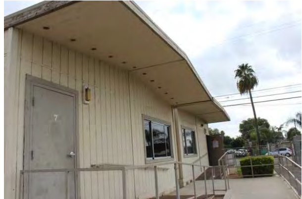
#32 LIGHT FIXTURE, EXTERIOR FLOOD
