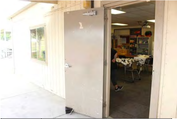
#13 EXTERIOR DOOR, STEEL
