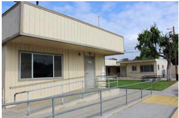
#12 EXTERIOR WALL WOOD SIDING
