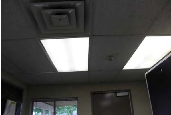
#19 INTERIOR CEILING FINISH, SUSPENDED ACOUSTICAL TILE (ACT)
