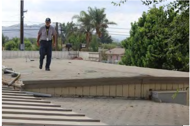
#14 ROOF, MODIFIED BITUMINOUS
