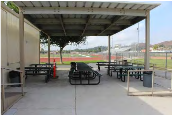
#11 ROOF STRUCTURE, FLAT, METAL DECK OVER STEEL BEAMS
