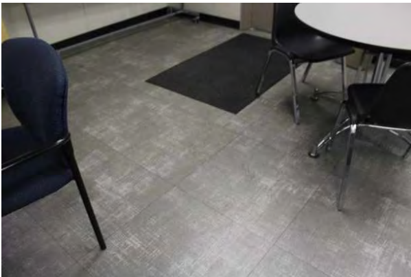
#17 INTERIOR FLOOR FINISH, VINYL TILE (VCT)
