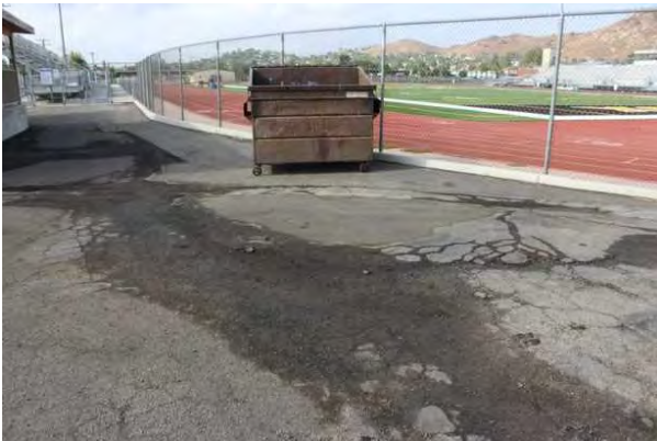
#39 PARKING LOTS, ASPHALT PAVEMENT
