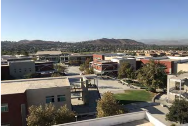
#7 CAMPUS ROOF OVERVIEW
