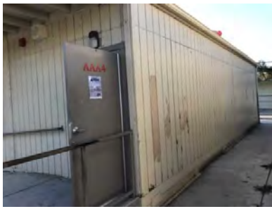
Damaged paint surface - AssetCALC ID: 1471538
