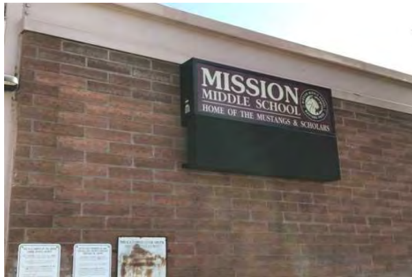
#7 PROPERTY BUILDING MOUNTED SIGNAGE
