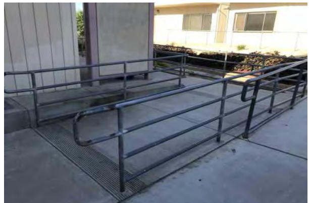
#66 EXTERIOR RAMP W/ RAILING
