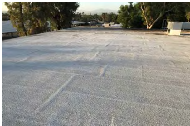
#12 MODIFIED BITUMINOUS ROOFING
