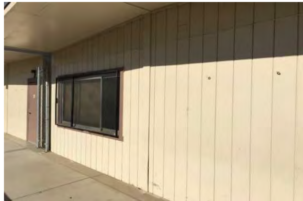
#8 EXTERIOR METAL DOOR, WOOD FACADE
