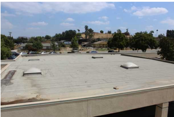
#17 ROOF, MODIFIED BITUMINOUS
