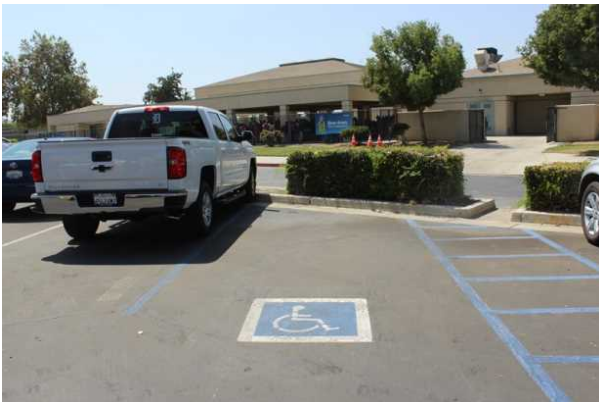
#59 PARKING LOTS, ASPHALT PAVEMENT
