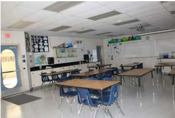
#23 INTERIOR FLOOR FINISH, VINYL TILE (VCT)
