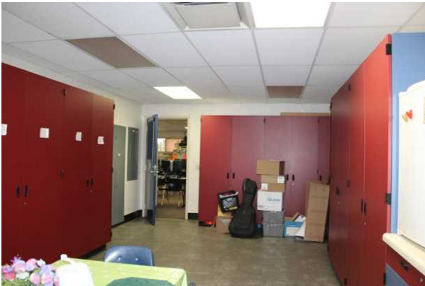
#21 INTERIOR FLOOR FINISH, VINYL TILE (VCT)
