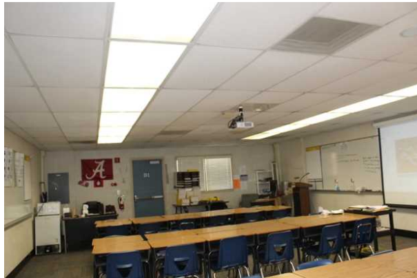
#28 INTERIOR CEILING FINISH, SUSPENDED ACOUSTICAL TILE FIBERGLASS (ACT)
