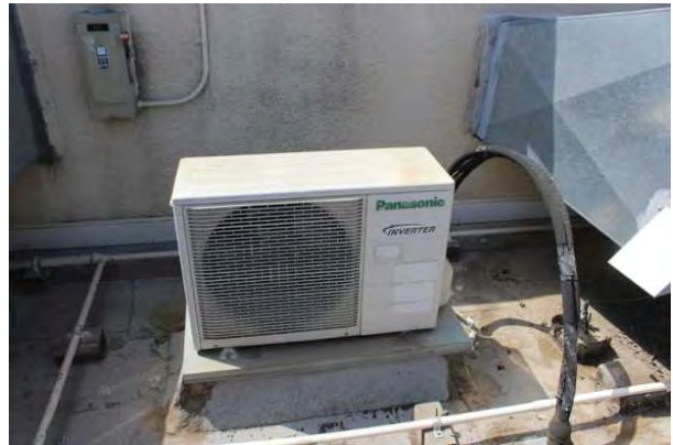
#40 DUCTLESS SPLIT SYSTEM, SINGLE ZONE
