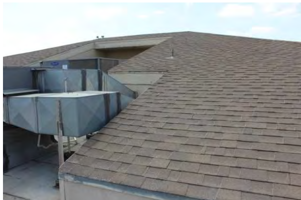
#16 ROOF, ASPHALT SHINGLE
