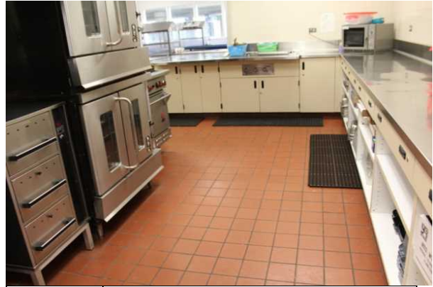
#20 INTERIOR FLOOR FINISH, QUARRY TILE
