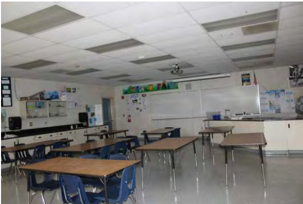
#27 INTERIOR CEILING FINISH, SUSPENDED ACOUSTICAL TILE FIBERGLASS (ACT)
