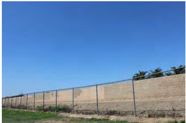
#60 FENCES AND GATES, CHAIN LINK
