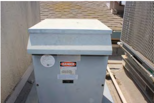
#47 SECONDARY TRANSFORMER
