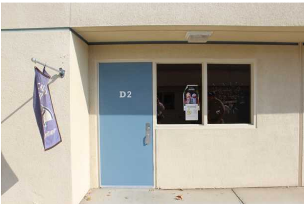
#15 EXTERIOR DOOR, STEEL
