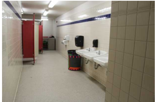
#22 INTERIOR FLOOR FINISH, CERAMIC TILE
