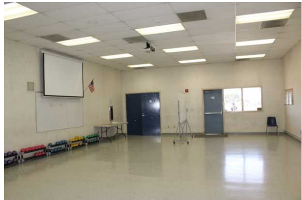
#24 INTERIOR FLOOR FINISH, LINOLEUM
