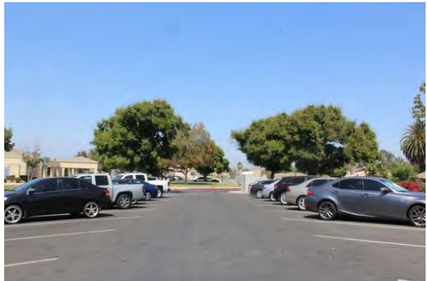
#58 PARKING LOTS, ASPHALT PAVEMENT
