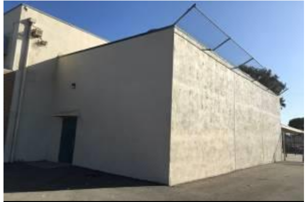
#50 EXTERIOR WALL, STUCCO
