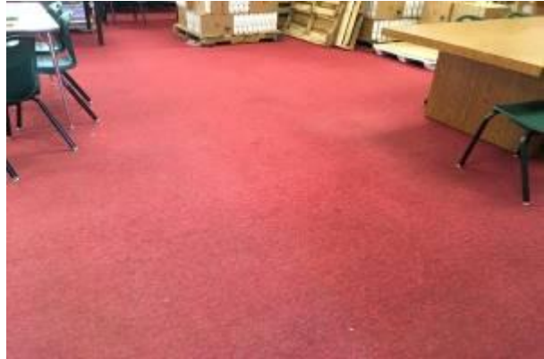
#38 INTERIOR FLOOR FINISH, CARPET
