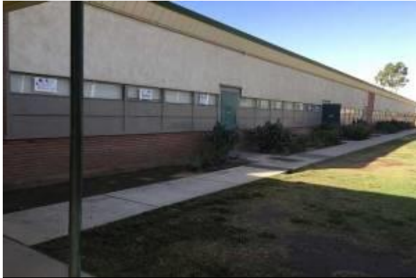
#7 NORH ELEVATION - BUILDING 300
