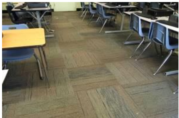
#36 INTERIOR FLOOR FINISH, CARPET
