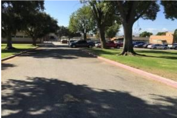
#21 PARKING LOTS, ASPHALT PAVEMENT
