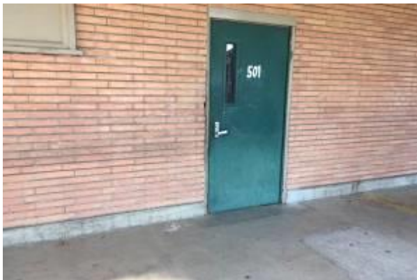
#33 EXTERIOR DOOR, STEEL,
