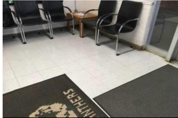
#44 INTERIOR FLOOR FINISH, VINYL TILE (VCT)
