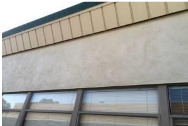
#53 EXTERIOR WALL, STUCCO
