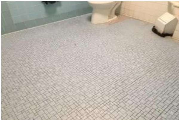
#45 INTERIOR FLOOR FINISH, CERAMIC TILE
