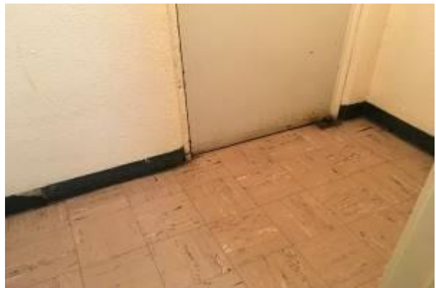
#54 INTERIOR FLOOR FINISH, VINYL TILE (VCT)
