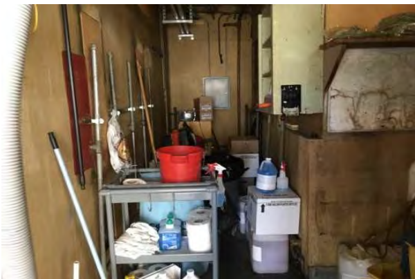
#41 C BUILDING UTILITY CLOSET
