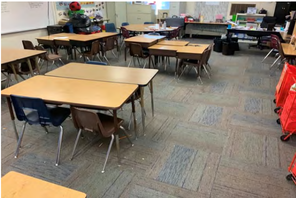
#27 INTERIOR FLOOR FINISH, CARPET TILE
