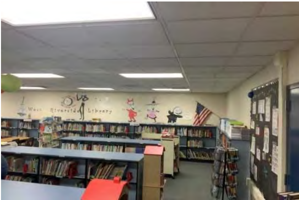
#21 LIGHTING SYSTEM, INTERIOR LIBRARY
