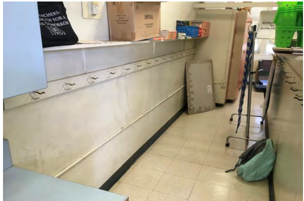
#28 INTERIOR WALL FINISH AND VCT TILE FLOORING
