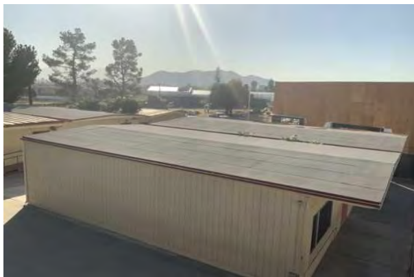
#42 PORTABLE ROOF ROLLED ASPHALT
