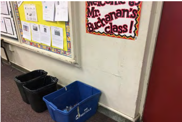
#29 INTERIOR WALL FINISH
