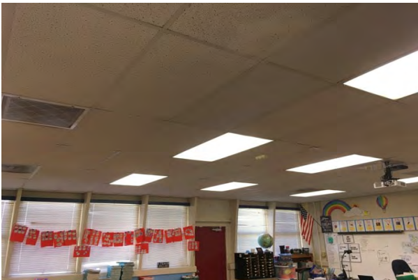
#23 INTERIOR CEILING FINISH, SUSPENDED ACOUSTICAL TILE (ACT)
