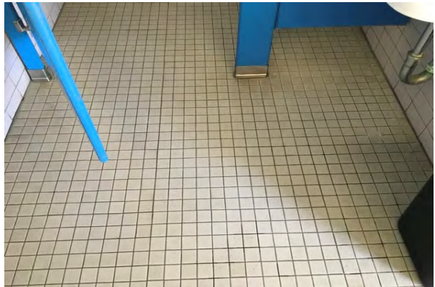
#34 INTERIOR FLOOR FINISH, CERAMIC TILE
