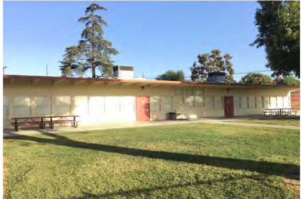
#2 A CLASSROOM BUILDING
