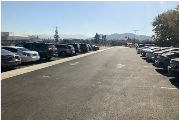
#51 PARKING LOTS, ASPHALT PAVEMENT, SEAL AND STRIPE
