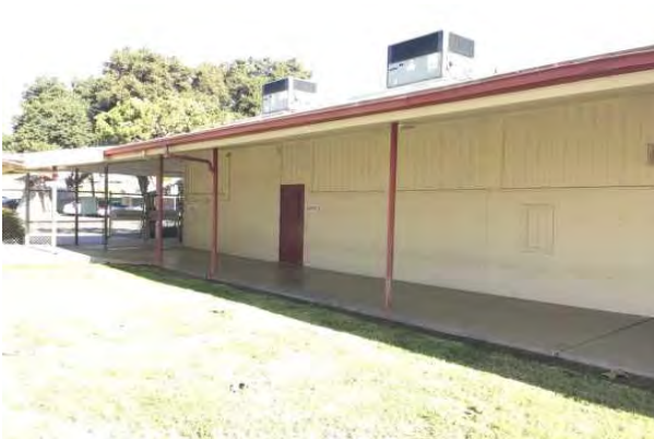
#5 J CLASSROOM BUILDING
