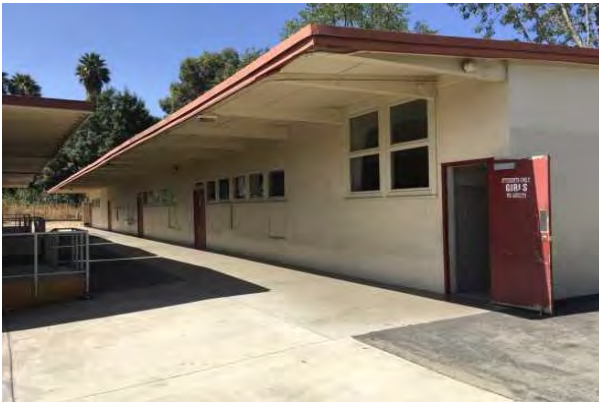
#9 G CLASSROOM BUILDING
