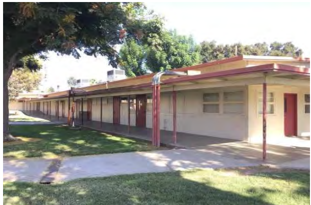
#6 C CLASSROOM BUILDING
