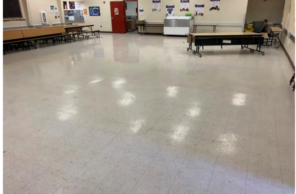
#26 INTERIOR FLOOR FINISH, VINYL TILE (VCT)
