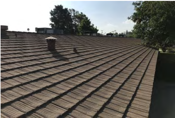
#27 BUILDING C ROOF
