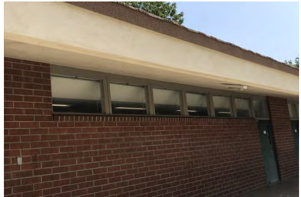
#34 BUILDING D WINDOWS
