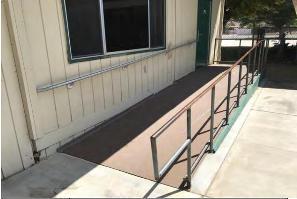
#19 PORTABLE EXTERIOR RAMP
