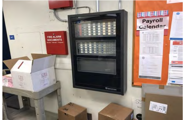
#50 BUILDING A FIRE ALARM PANEL
