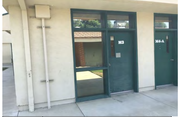
#32 BUILDING M EXTERIOR DOORS AND WINDOWS
