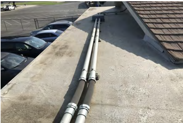
#29 ROOF AT WALKWAY
