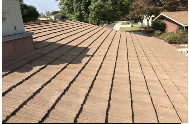
#26 BUILDING F ROOF
