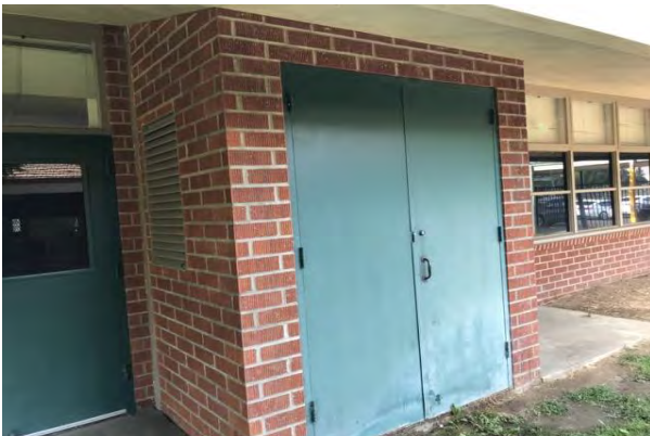
#35 BUILDING B EXTERIOR UTILITY DOOR
