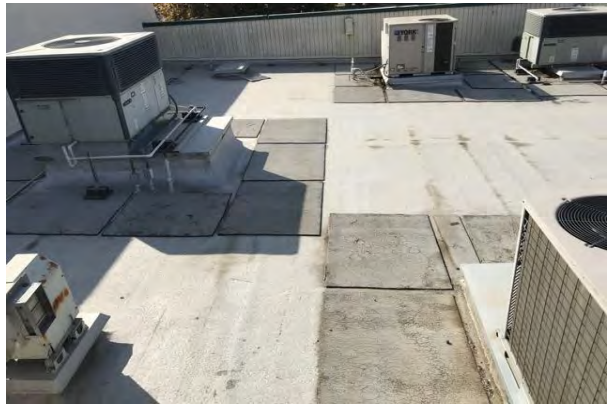
#28 ROOF, BUILT-UP AT BUILDING M
