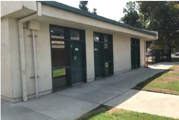
#33 BUILDING M EXTERIOR DOOR
