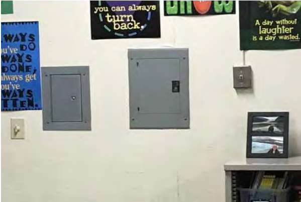
#49 PORTABLE MAIN DISTRIBUTION PANEL
