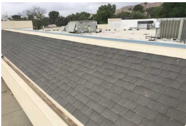
#23 PRIMARY ROOF OVERVIEW
