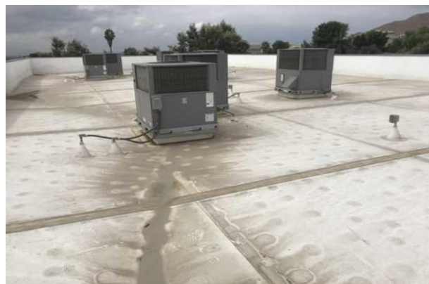
#24 SECONDARY ROOF OVERVIEW
