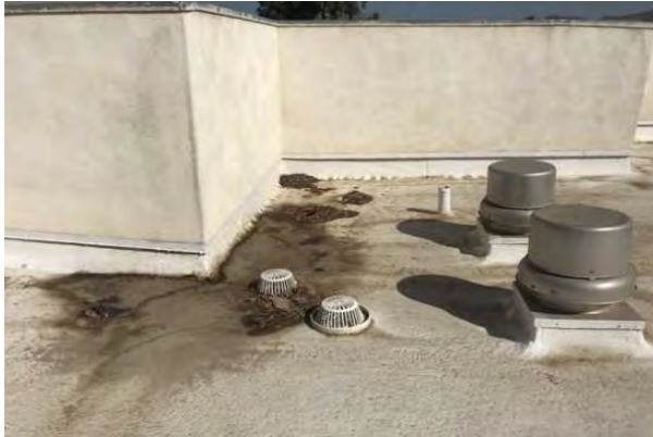
#25 DRAINAGE / PARAPET WALL EDGE / FLASHINGS
