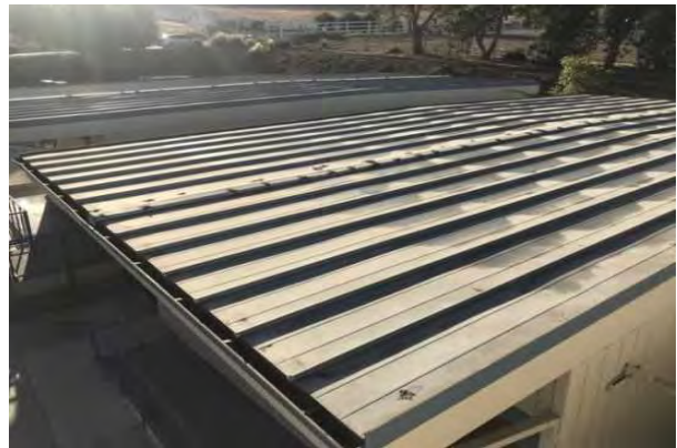
#24 METAL ROOF OVERVIEW
