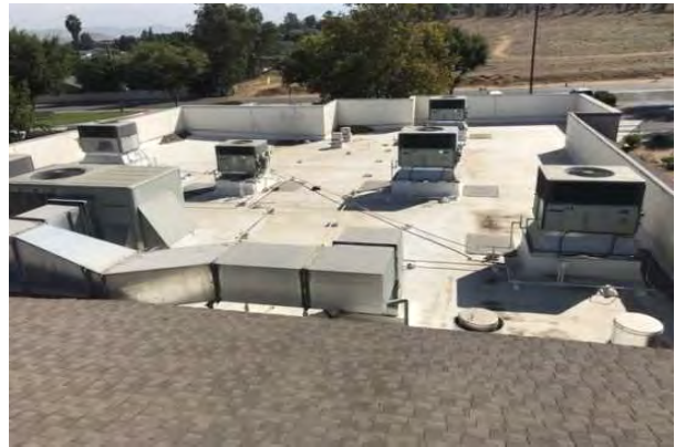
#22 PRIMARY ROOF OVERVIEW
