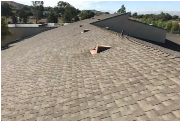
#23 SECONDARY ROOF OVERVIEW
