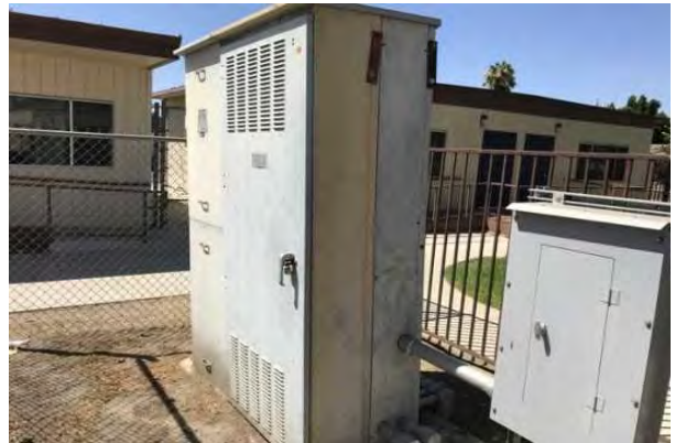
#10 BUILDING/MAIN SWITCHBOARD
