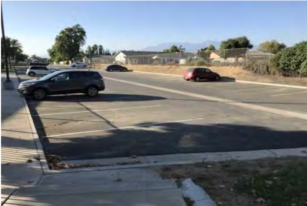
#7 PARKING LOT AND HARDSCAPE OVERVIEW
