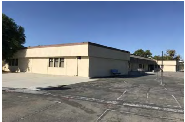
#16 OVERALL CLASSROOM BUILDING
