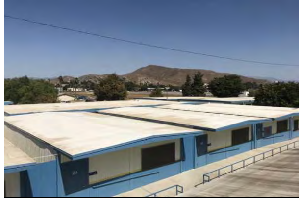
#26 SECONDARY ROOF OVERVIEW
