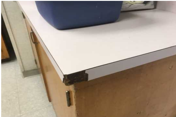
#45 DELAMINATING COUNTERTOPS
