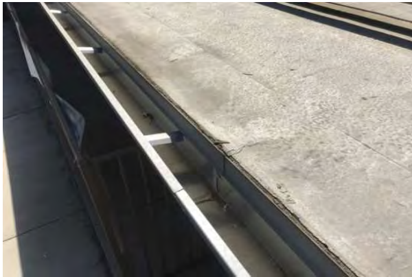
#27 DRAINAGE / PARAPET WALL EDGE / FLASHINGS
