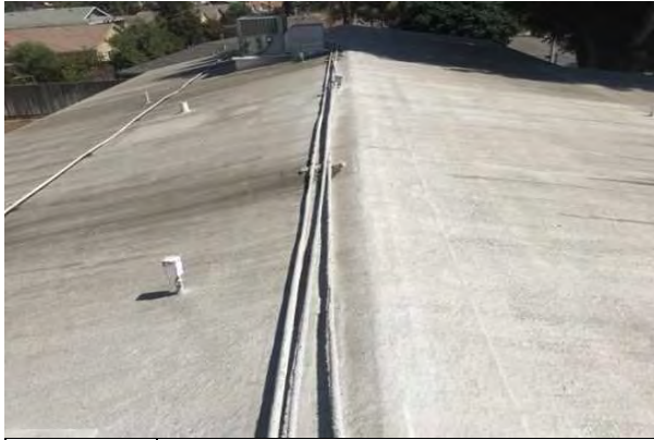
#25 PRIMARY ROOF OVERVIEW
