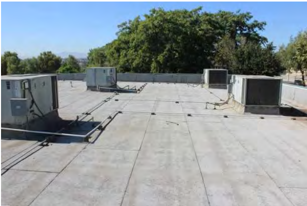
#15 ROOF, MODIFIED BITUMINOUS
