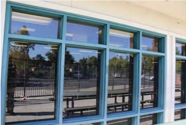
#13 STOREFRONT, METAL-FRAMED WINDOWS
