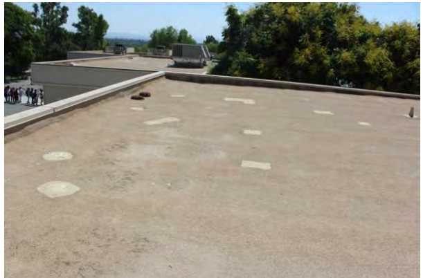
#10 ROOF POLYURETHANE COATING
