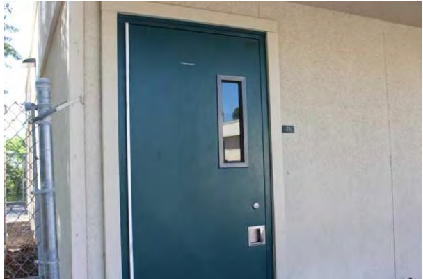
#14 EXTERIOR DOOR, STEEL
