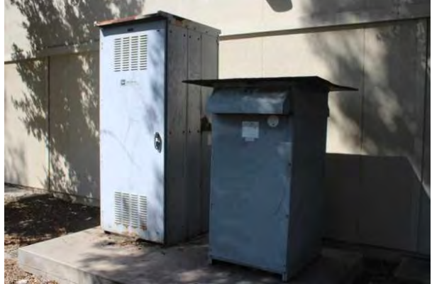
#38 SECONDARY TRANSFORMER
