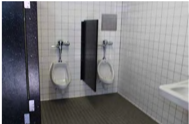
#18 INTERIOR FLOOR FINISH, CERAMIC TILE
