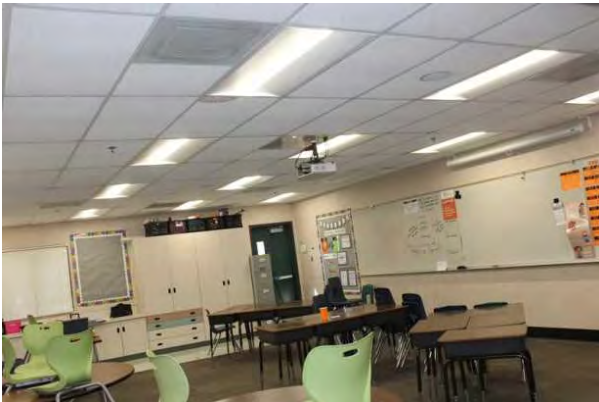
#21 INTERIOR CEILING FINISH, SUSPENDED ACOUSTICAL TILE (ACT)
