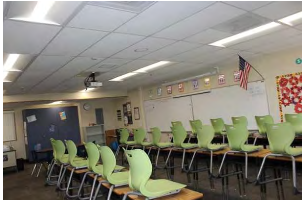
#22 INTERIOR CEILING FINISH, SUSPENDED ACOUSTICAL TILE (ACT)
