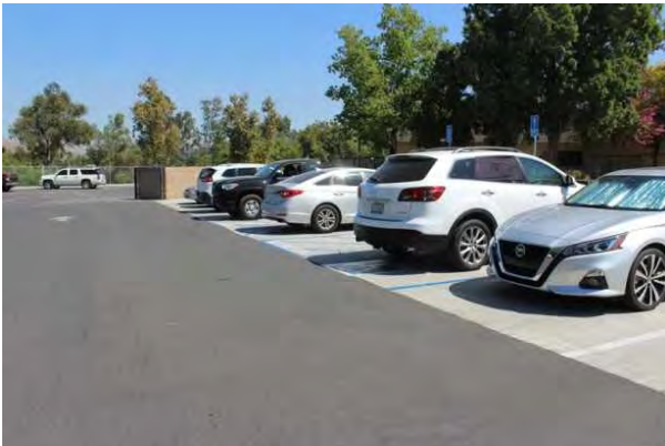
#51 PARKING LOTS, ASPHALT PAVEMENT
