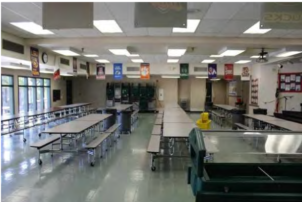
#17 INTERIOR FLOOR FINISH, VINYL TILE (VCT)
