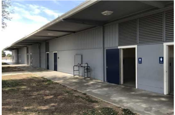
#2 CLASSROOMS BUILDING EXTERIOR
