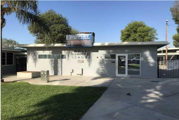
#1 ADMINISTRATION BUILDING EXTERIOR
