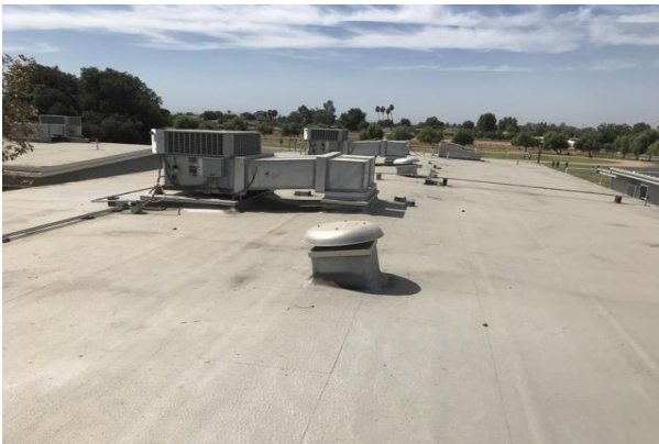
#23 CLASSROOMS BUILDINGS ROOF
