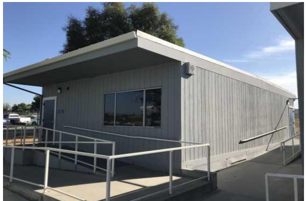
#6 PORTABLE CLASSROOM EXTERIOR
