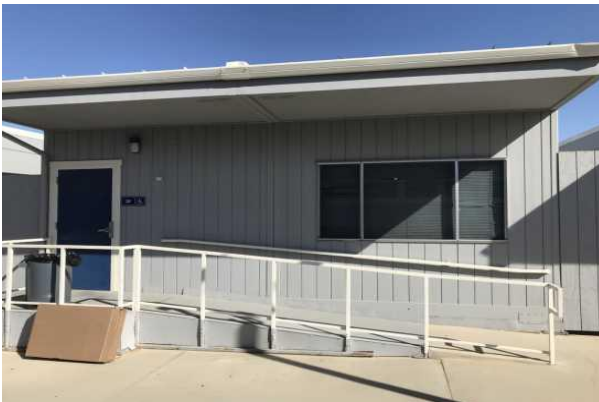
#5 PORTABLE CLASSROOM EXTERIOR
