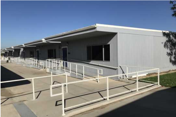
#7 PORTABLE CLASSROOM EXTERIOR
