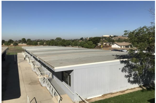
#22 PORTABLE CLASSROOMS ROOFS
