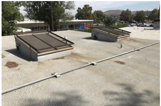
#24 CLASSROOMS BUILDINGS ROOF - SKYLIGHTS
