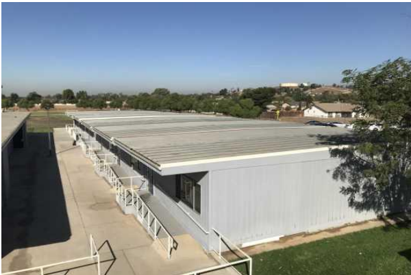
#9 PORTABLE CLASSROOM EXTERIOR
