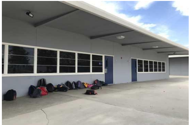
#4 CLASSROOMS BUILDING EXTERIOR
