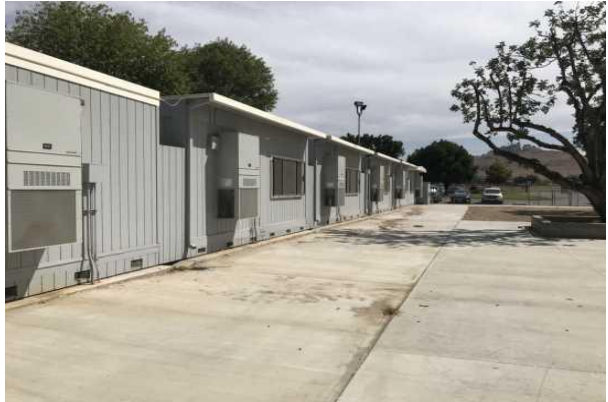
#8 PORTABLE CLASSROOM EXTERIOR
