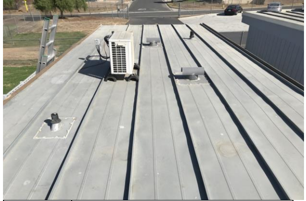
#26 RESTROOMS BUILDING ROOF
