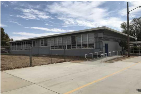
#3 CLASSROOMS BUILDING EXTERIOR
