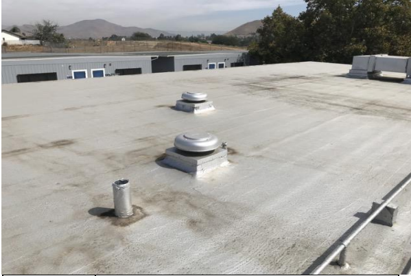
#25 CLASSROOMS BUILDINGS ROOF
