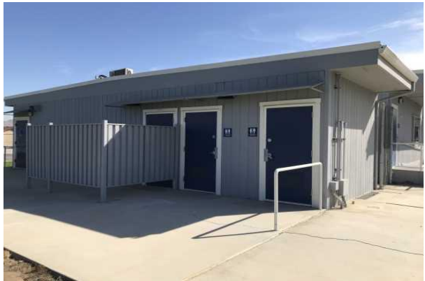
#10 RESTROOM BUILDING EXTERIOR
