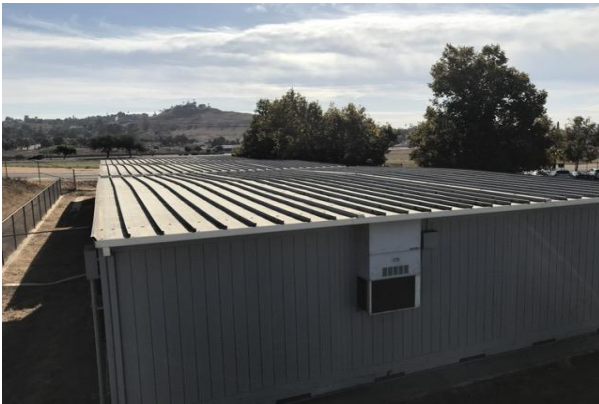
#21 PORTABLE CLASSROOMS ROOFS
