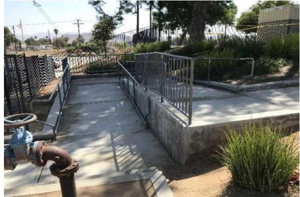
#50 EXTERIOR CONCRETE RAMP WITH HAND-RAILING
