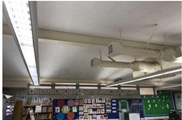
#52 HARD TILE CEILING, HVAC DUCTWORK
