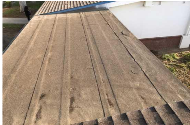
#10 MODIFIED BITUMINOUS ROOFING
