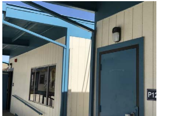
#48 EXTERIOR METAL DOOR, METAL FRAME WINDOW
