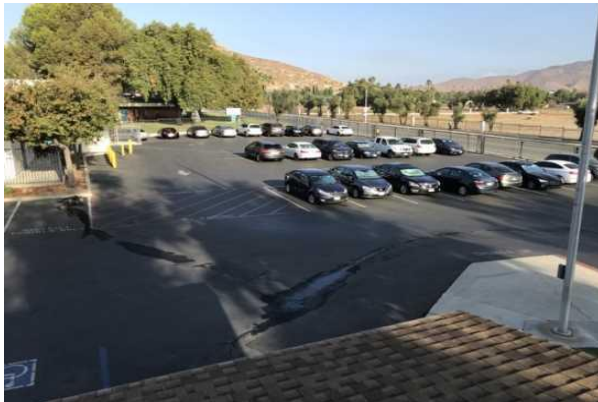
#51 ASPHALT PARKING LOT
