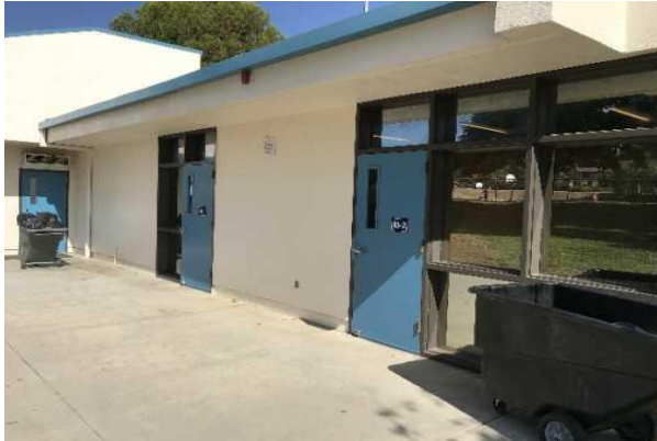
#7 STUCCO FACADE, EXTERIOR METAL DOOR
