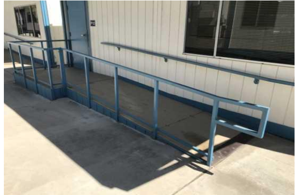
#8 EXTERIOR RAMP, WOOD FACADE
