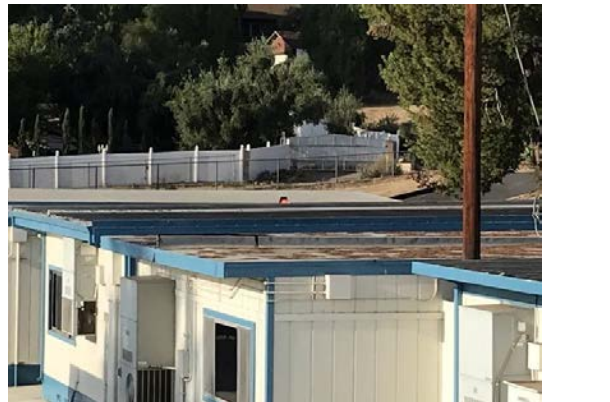
#12 MODIFIED BITUMINOUS ROOFING
