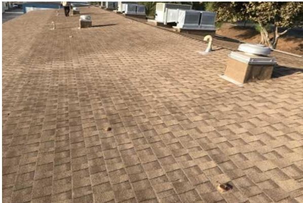
#9 ASPHALT SHINGLE ROOFING
