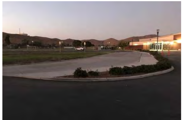
#6 PARKING LOT AND HARDSCAPE OVERVIEW
