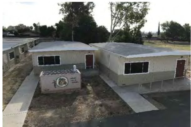
#10 MODIFIED BITUMINOUS ROOFING, PORTABLE BUILDINGS
