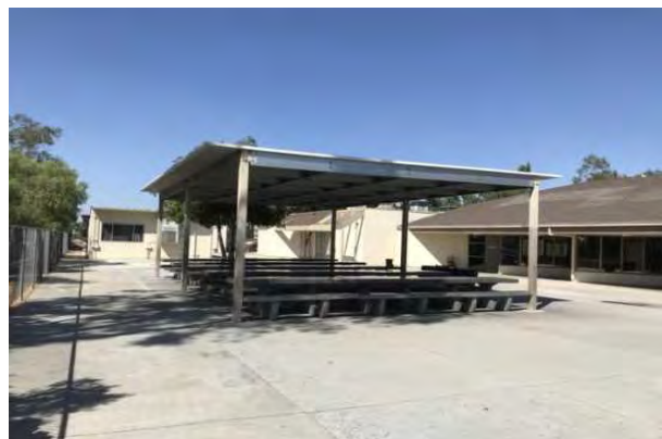
#42 METAL CANOPY STRUCTURE
