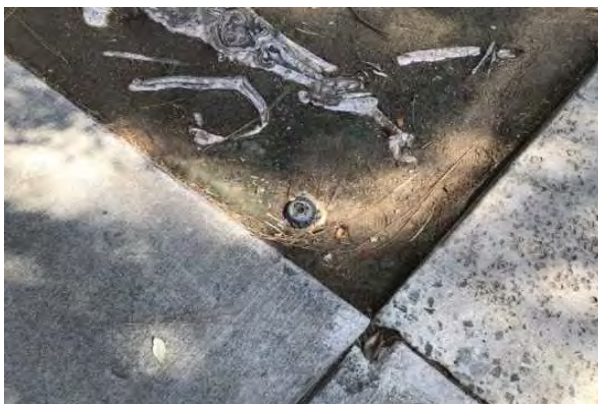
#41 SITE IRRIGATION SYSTEM
