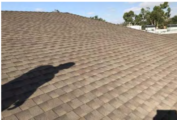
#9 ASPHALT SHINGLE ROOFING
