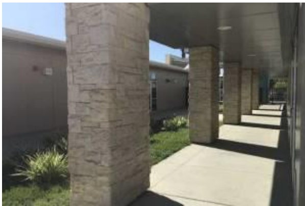
#15 EXTERIOR WALL, STONE VENEER
