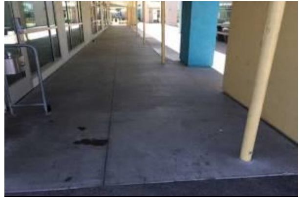
#38 PEDESTRIAN PAVEMENT, SIDEWALK
