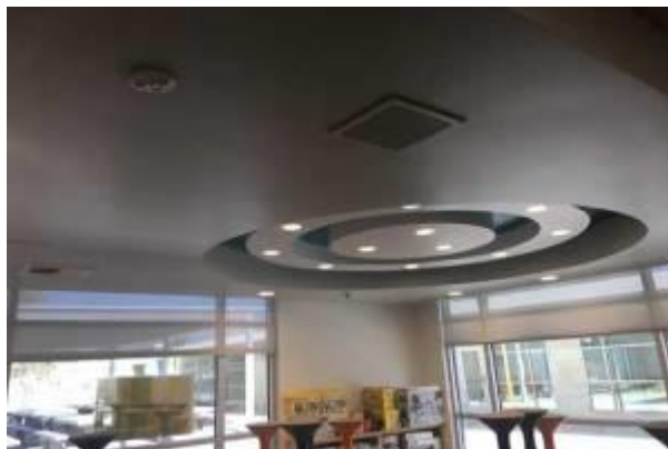
#23 INTERIOR CEILING FINISH
