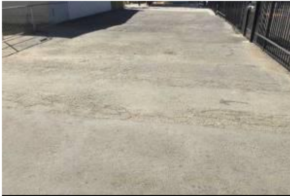
#37 PARKING LOTS, ASPHALT PAVEMENT
