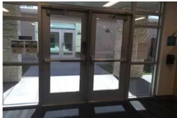
#16 EXTERIOR DOOR, ALUMINUM-FRAMED FULLY-GLAZED
