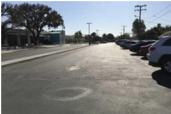
#35 PARKING LOTS, ASPHALT PAVEMENT
