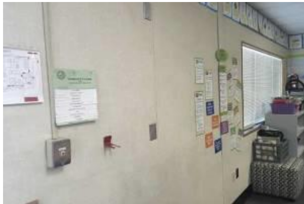
#19 INTERIOR WALL CONSTRUCTION, FIBERGLASS PANEL
