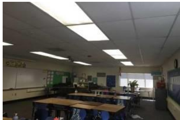
#24 INTERIOR CEILING FINISH
