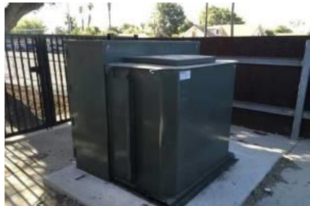
#28 SECONDARY TRANSFORMER
