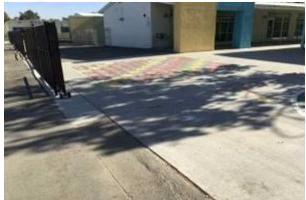
#36 PARKING LOTS, CONCRETE PAVEMENT
