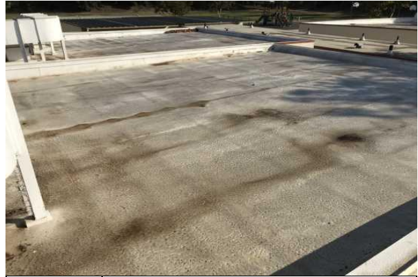
#8 SINGLE-PLY TPO/PVC ROOFING
