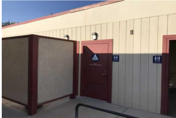
#13 EXTERIOR METAL DOOR, WOOD SHINGLE
