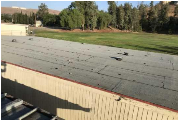
#9 MODIFIED BITUMINOUS ROOFING
