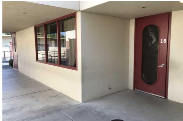
#12 STUCCO FACADE, EXTERIOR METAL PARTIALLY GLAZED DOOR
