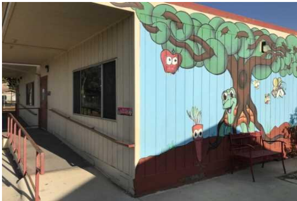
#11 WOOD FACADE, METAL WINDOW
