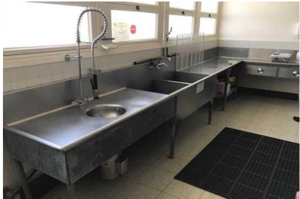
#34 MPR BUILDING KITCHEN - SINKS
