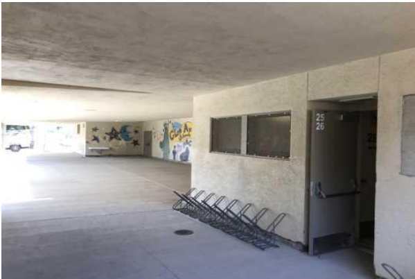
#27 MBR BUILDING - EXTERIOR
