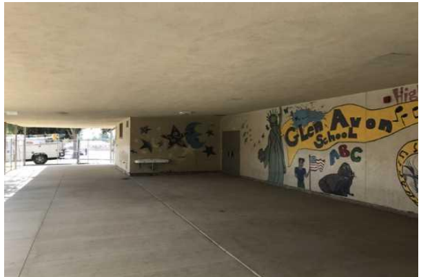
#28 MBR BUILDING - EXTERIOR
