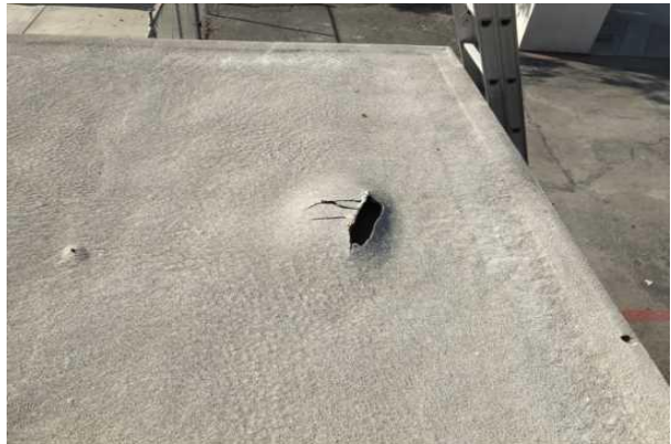
#22 MPR BUILDING ROOF
