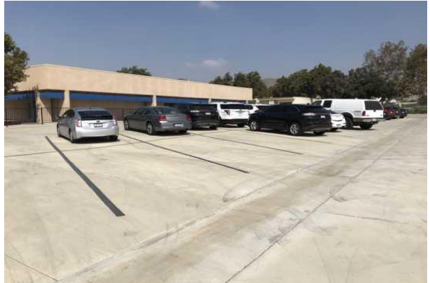
#8 REAR PARKING LOT
