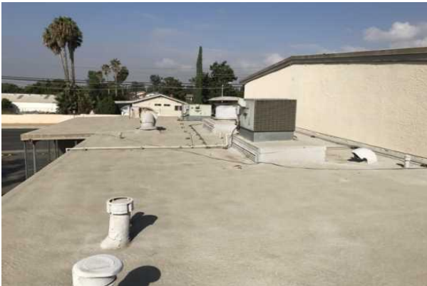
#21 MPR BUILDING ROOF
