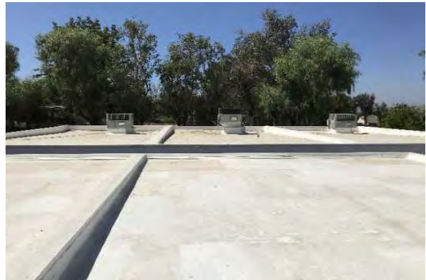
#10 SINGLE-PLY TPO/PVC ROOFING
