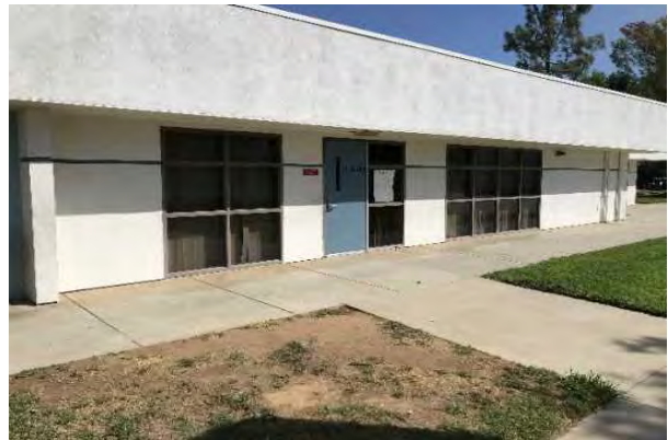
#6 STUCCO FACADE, METAL FRAME WINDOW, EXTERIOR METAL PARTIALLY GLAZED DOOR
