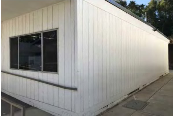
#7 WOOD FACADE, METAL SINGLE-PANE WINDOW
