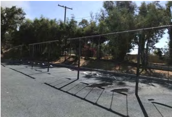
#45 PLAYGROUND SWING, DETERIORATING RUBBER SURFACE
