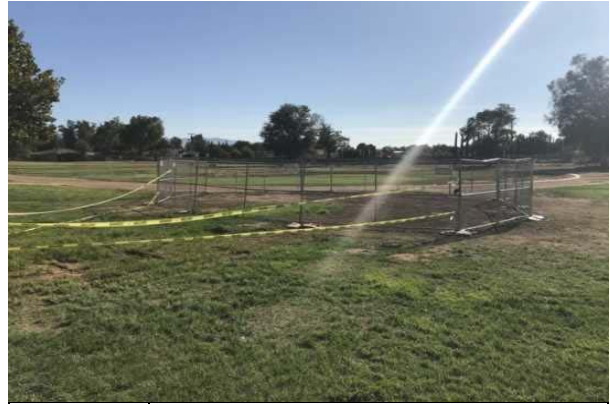
#44 AREA OF STORMWATER DRAINAGE DAMAGE
