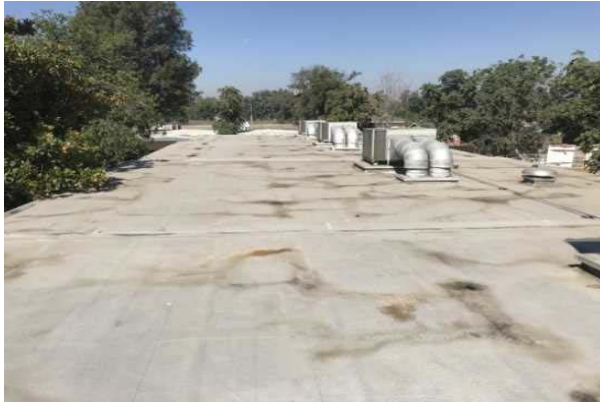
#21 MODIFIED BITUMEN ROOFING
