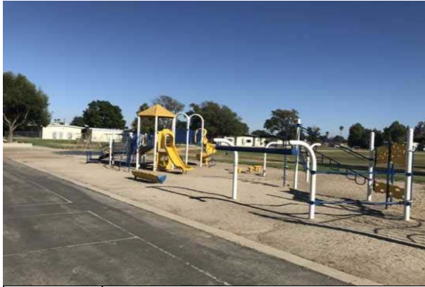
#43 NO ADA ACCESS TO PLAY STRUCTURES
