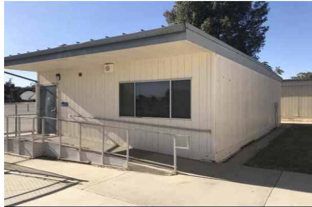
#6 MODULAR CLASSROOM BUILDING
