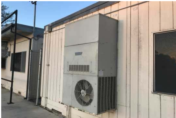
#29 WALL-MOUNTED HEAT PUMP
