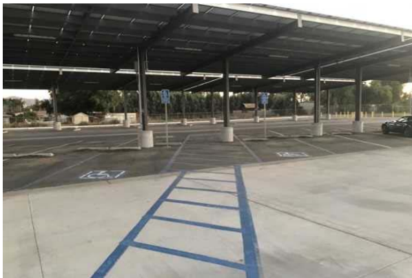
#39 PAVEMENT AND CARPORT STRUCTURES
