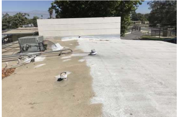
#22 SPRAY POLYURETHANE FOAM ROOFING
