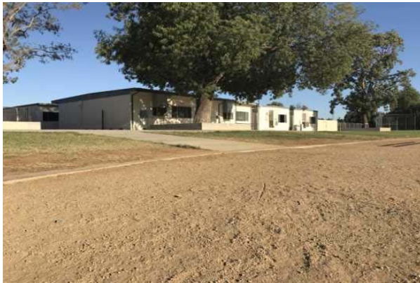
#45 SLOPE OF WALKWAY/RAMP TO TRACK NOT ADA ACCESSIBLE
